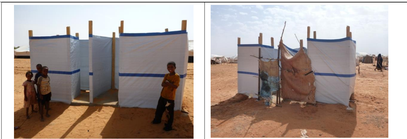
Figure – Emergency Showers where users installed their own privacy barrier
