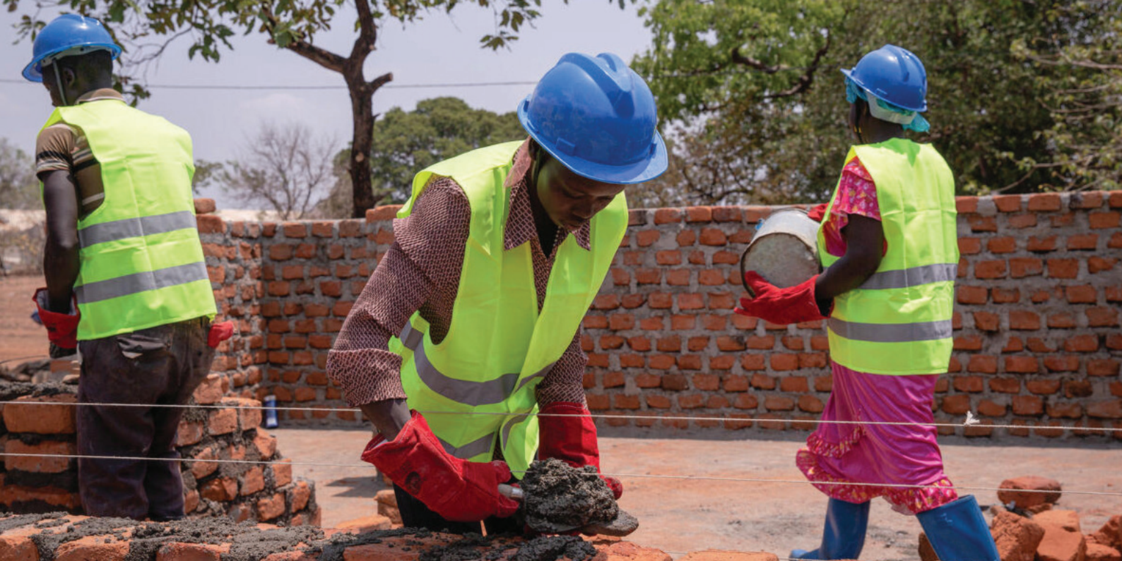
© UNHCR/Esther Ruth Mbabazi. South Sudanese refugee working in construction at the Bidibidi settlement in Uganda.
