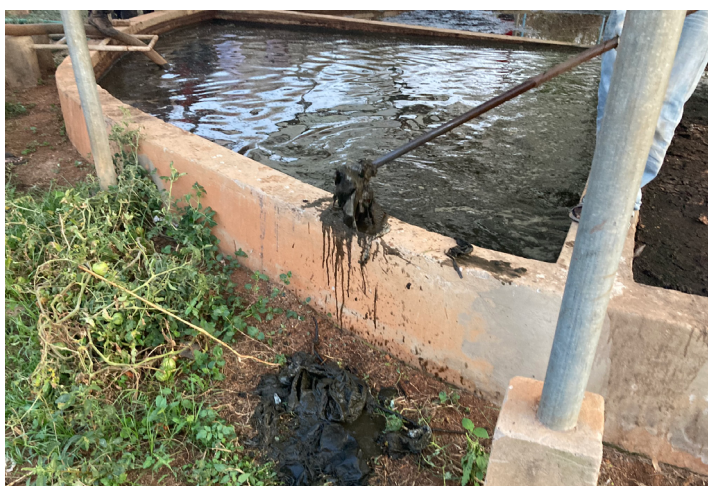
Figure 9: A treatment plant operator removing solid waste with a trash hook (source: Eawag).
