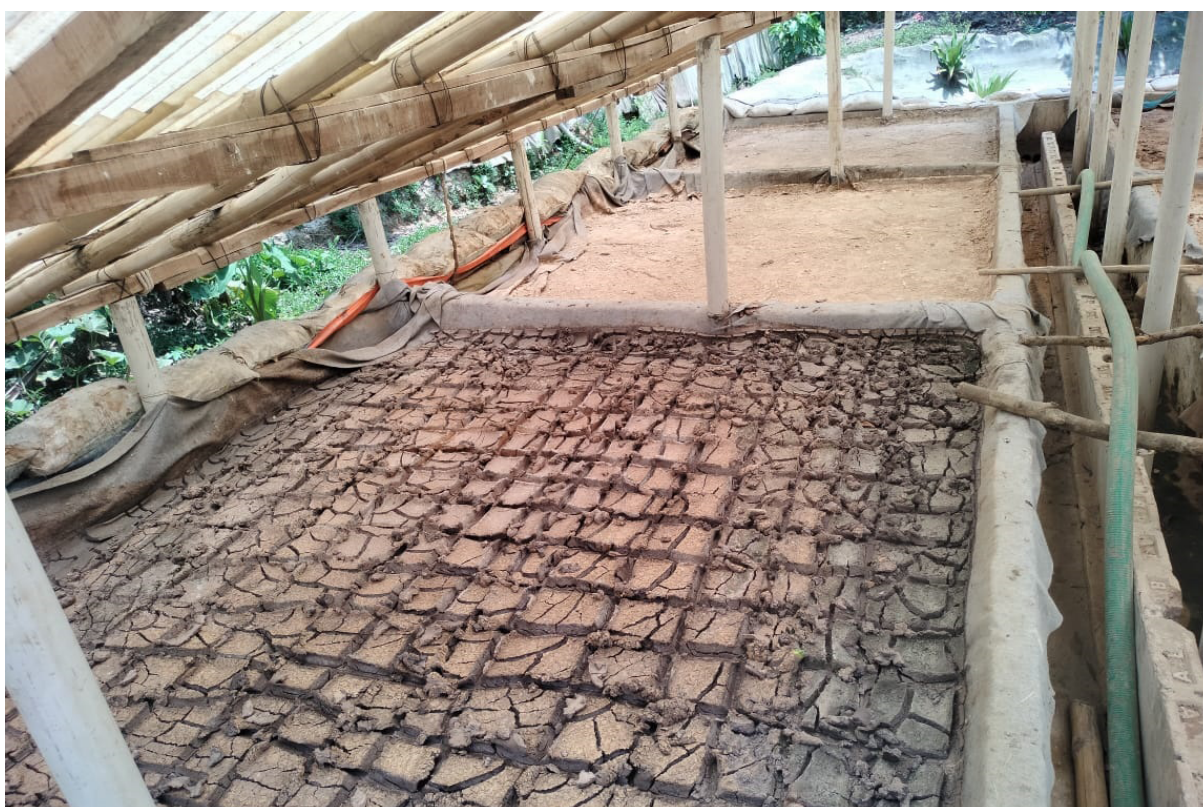
Figure 15: An unplanted drying bed loaded with faecal sludge in Cox's Bazar, Bangladesh (source: UNHCR).
